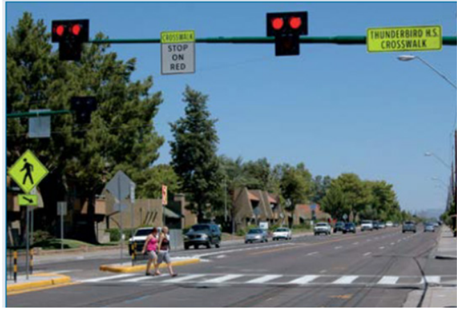
Pedestrian Hybrid Beacon (PHB) (Source: FHWA)
