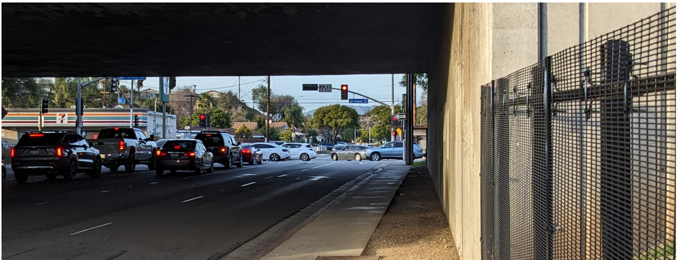
Wilcox Avenue underpass
